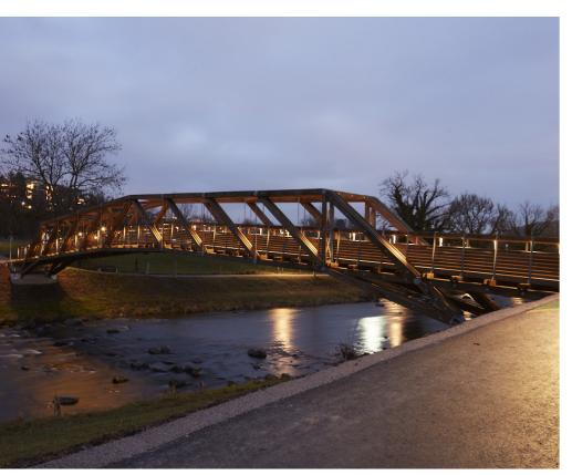
The Tüfisteg pedestrian and bicycle bridge in Adliswil was getting on in years. Renovating the lattice bridge would have cost almost as much as replacing it. It was obvious, therefore, that the bridge should be rebuilt. Beech wood from the region was used.
