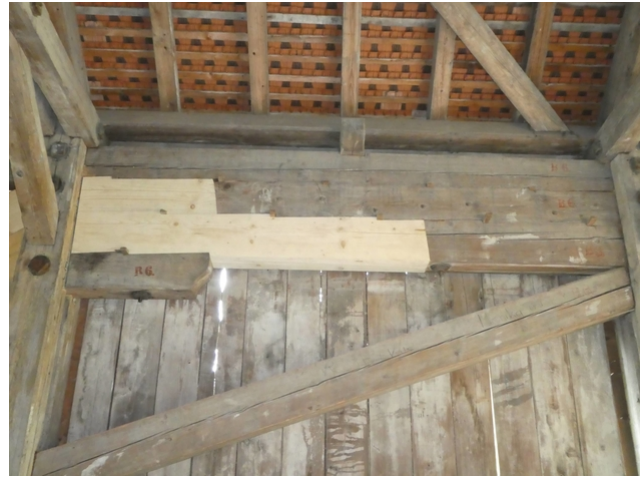
Existing and refurbished structure
