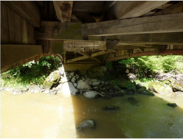
Bottom view of the bridge
