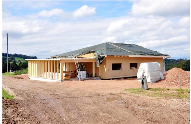
The rurally located single-family house was completely prefabricated and after only 4 months of construction the building was ready for occupancy. The timber construction contains a world novelty - namely the TS 3.0 developed by Timbatec - a ceiling system made of panels, which carry 2-axes analogous to a concrete ceiling.
