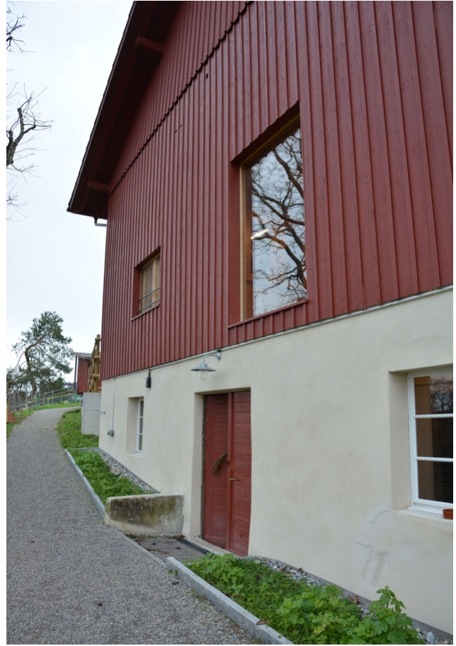
Red painted facade
