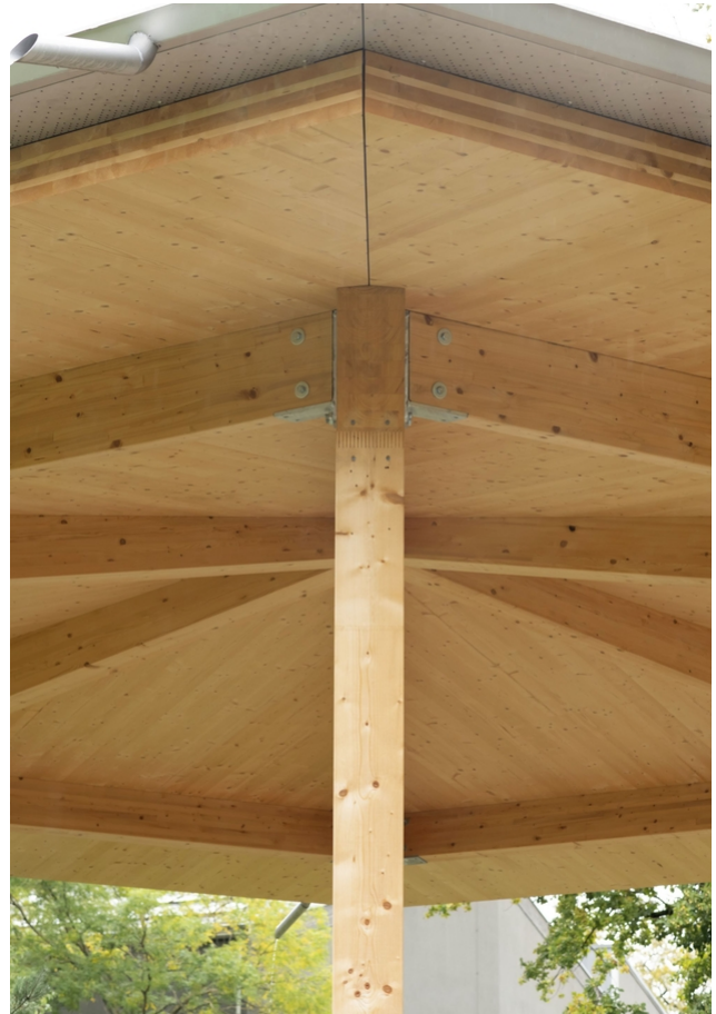
View of corner posts including beam connections
