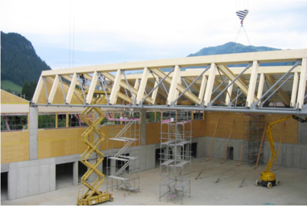
Assembly of lattice girders
