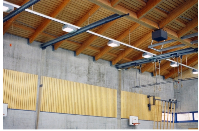
View of exposed rafter position
