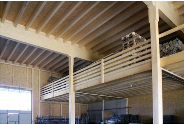
Storage space in the gallery area
