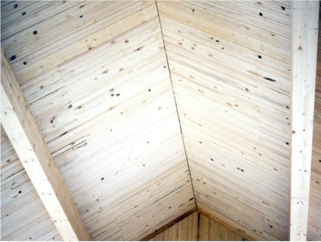
Roof construction with optiholz board stack modules
