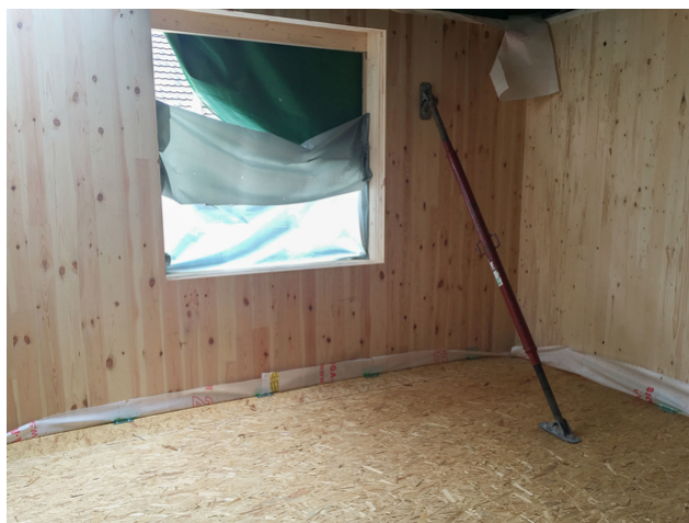
During the construction work: Load-bearing exterior walls made of solid wood
