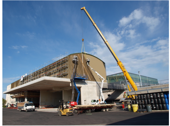
Assembly facade elements
