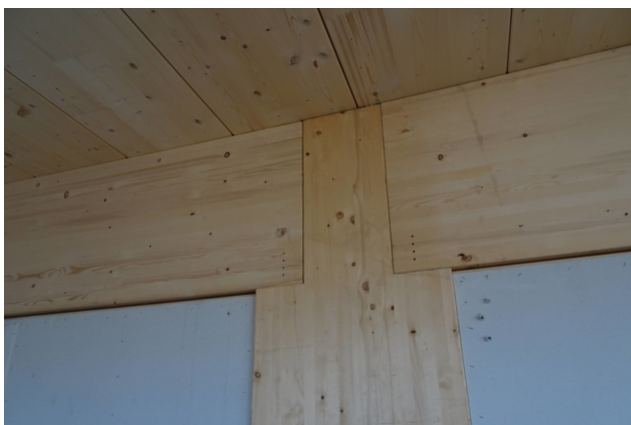
Bearing of the beams on the supports
