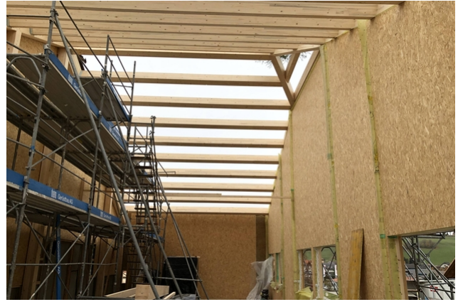
Extension gable side
