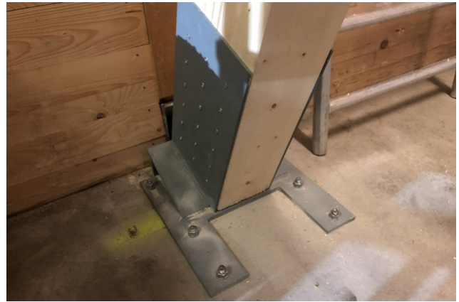
Strut connection bottom
