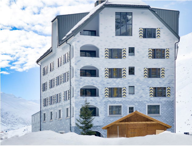
Heavy-duty roofs: Timbatec planned the roof structures
